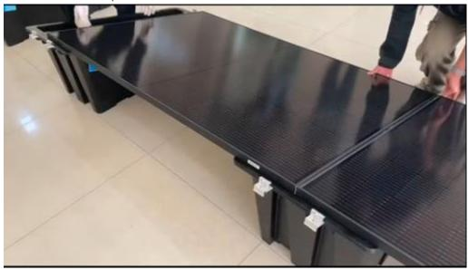
9. After confirming the position of the solar panel, tighten the screws on the clamps to fix it.
